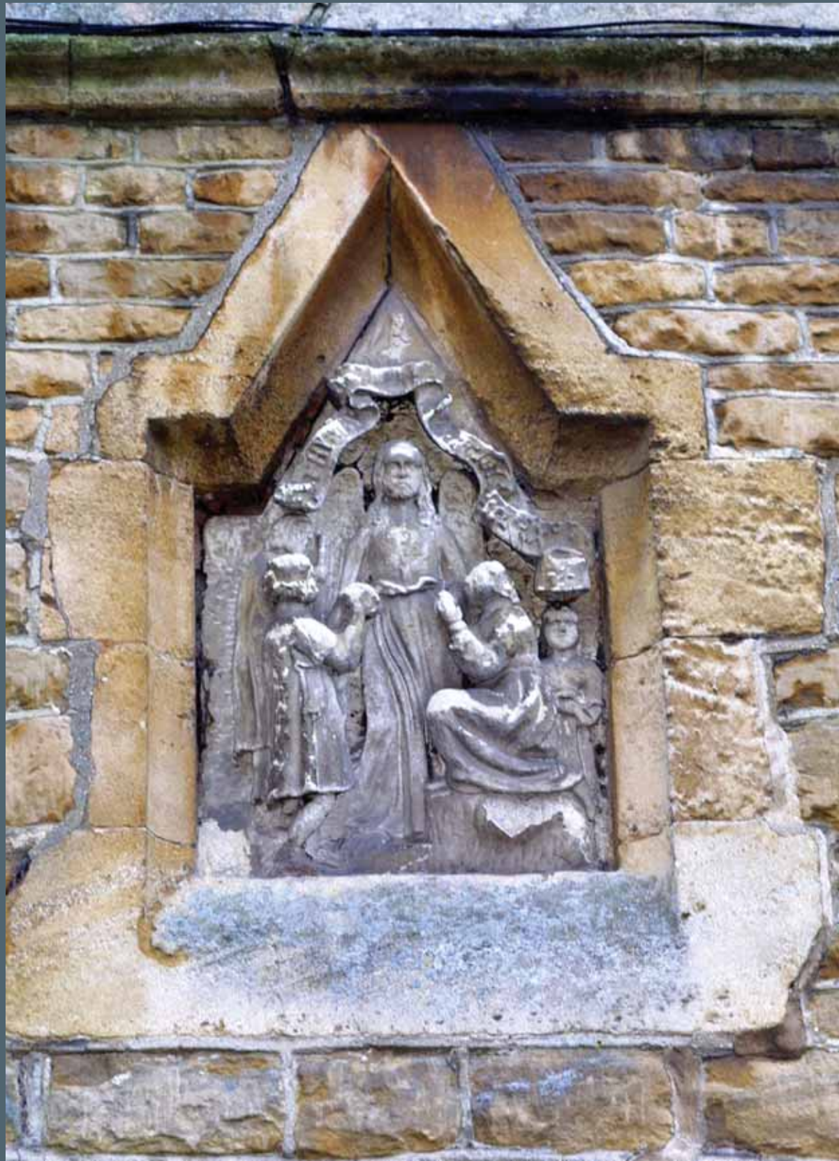
Detail from Receiving Office wall
